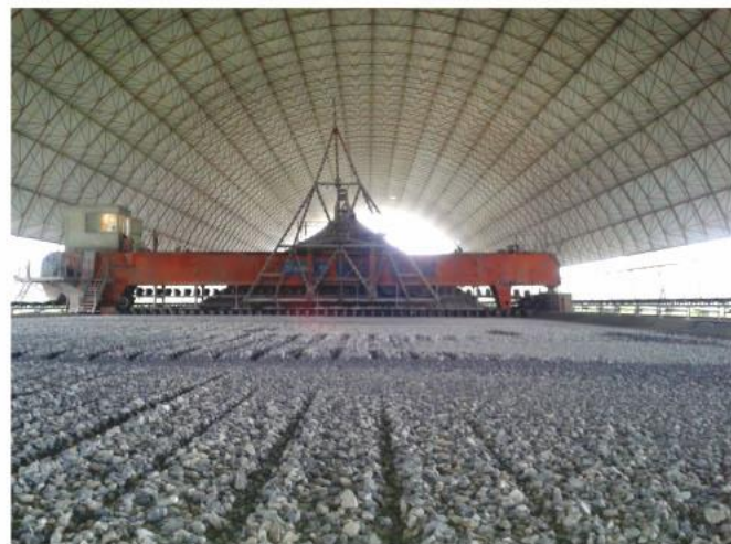
▲ Advanced homogenization system for raw materials
